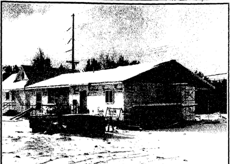
Despite the frigid weather the past few weeks, work has been continuing at the new house being built by Habitat for Humanity HiawathaLand at Fifth and Badger streets in Manistique. Delta-Schoolcraft ISD building trades students have been installing insulation and recently began hanging drywall. While the house looks similar to other Habitat homes, this project is a different, as the building will be completely wheelchair accessible. Outside ramps will allow safe access. Inside, the bathroom will have both a regular bath/shower and a wheelchair-accessible shower. Also, thermostats and cupboards will be placed lower for easier access and use. (Submitted photo)
