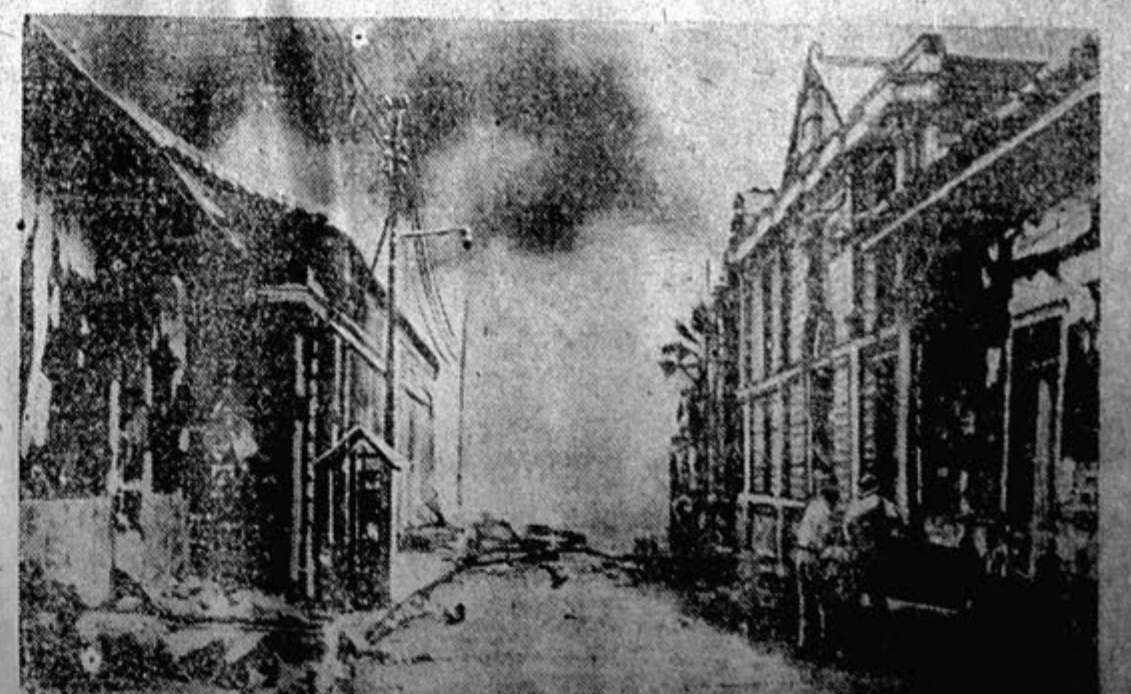
EARTHQUAKE HORROR IN HONDURAS —One of the year's biggest disasters was the earthquake in Honduras which practically destroyed Managua, the capital, killing an estimated 100,000 people. Smoldering ruins are shown here as a fire added to the destruction.
