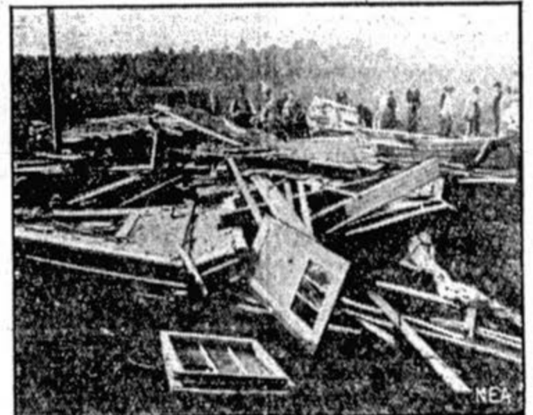
As Arkansas Tornado Struck
