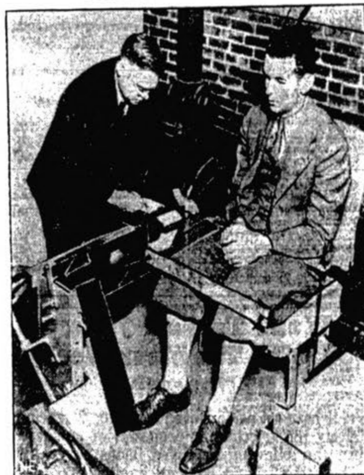
Life is just one jolt after another at Purdue University these days, and here you see M. F. White, graduate student, being "taken for a ride" on the Indiana school's new "shake table." Professor H. M. Jacklin, professor of automotive engineering, who designed the table to test the relative effects of different kinds of upholstery on the comfort of auto passengers, is shown at the left checking the recording instruments. Hands stretched across the knees and thighs of the riders record the extent to which comfortable posture is lost.
