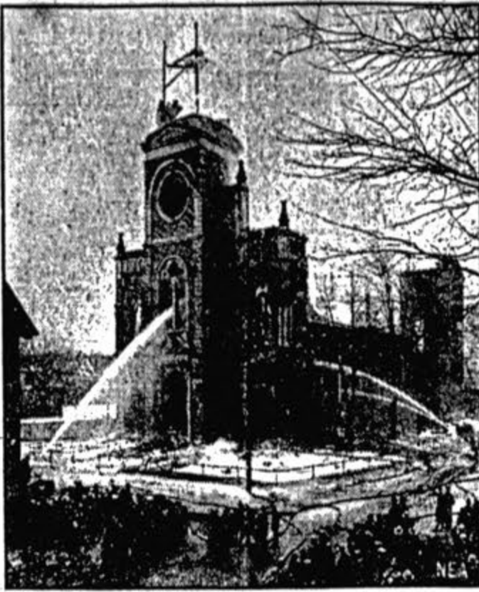
A candle in St. Joseph's Roman Catholic church at Ottawa, Ont., was upset accidentally by a parishioner who was praying the other day. The candle started a fire that set the whole church ablaze, and the building was almost completely destroyed, with a loss of $450,000. This picture shows firemen struggling with the flames.
