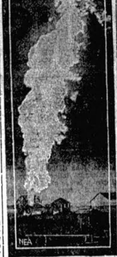
Here's a scene that proves bringing in a gas well isn't always profitable. This one, near Oklahoma City, caught fire as it blew in, and caused a loss of approximately $50,000 to its owners before the blaze was extinguished by "shots" of 200 pounds of nitroglycerine.
