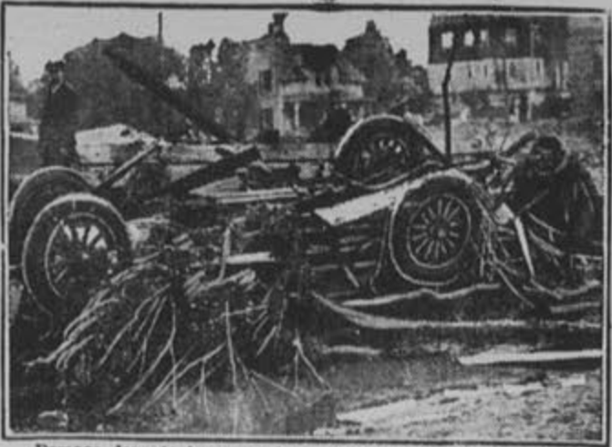
Damage done to houses and to the Boston & Maine Railroad at Willimansett, Mass., when two dams broke is estimated at $1,000,000. The dam of Langwald Pond burst. When the water swept into Robert's Pond below, that dam collapsed. The overturned auto shows the force of the water.
