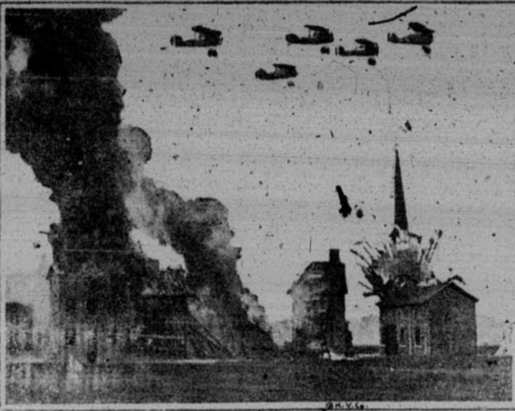
This village was constructed in England for a demonstration of the advances made in aerial warfare. Most of the buildings were made of spare airplane parts. The church steeple is 40 feet high. All of the men who took part in the bombing were veterans of the World War. When they finished—
