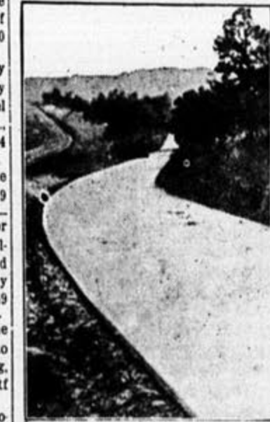
Concrete Road in Suburbs of Chicago.
