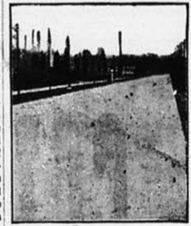
Experimental Concrete Road.
