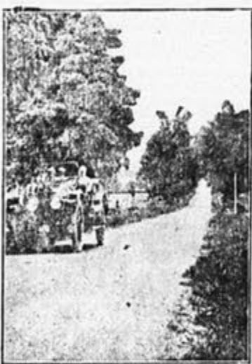
New Jersey State Road, Bituminous Macadam.
