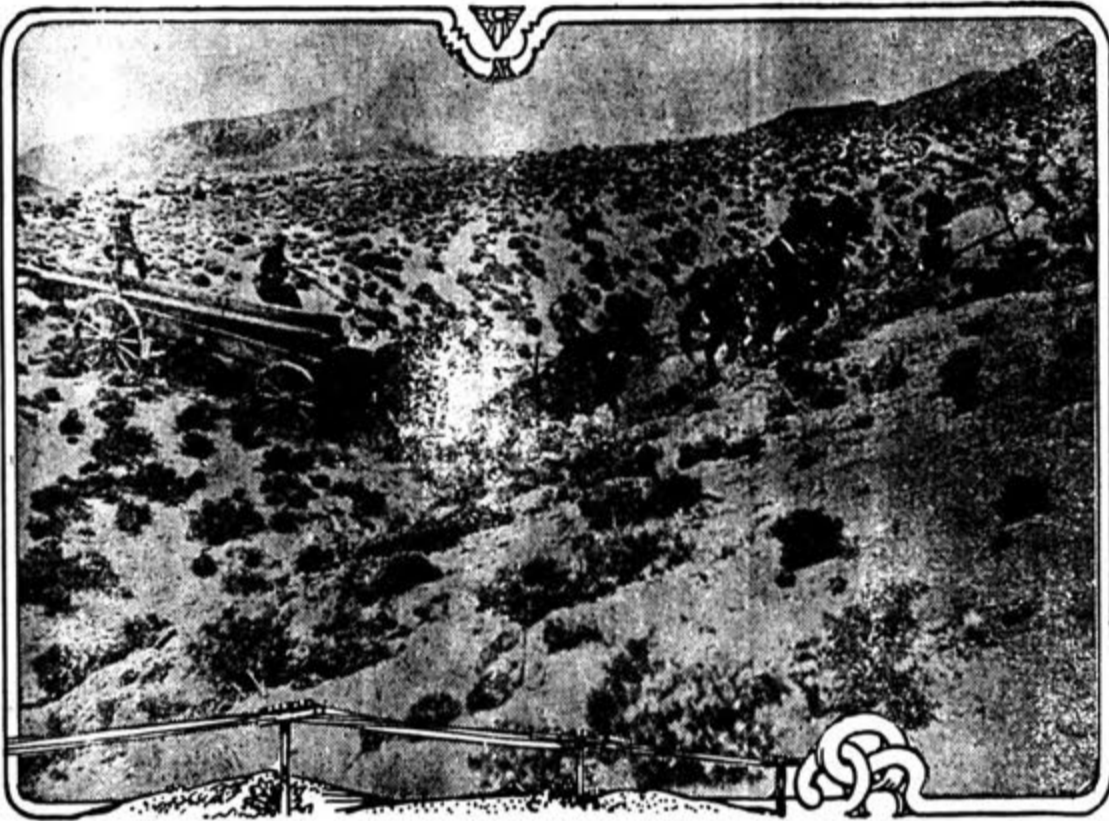
THE ABOVE PICTURE SHOWS THE TREMENDOUS DIFFICULTIES ENCOUNTERED IN CONSTRUCTING THE TRANSCONTINENTAL TELEPHONE LINE. IN MANY PLACES THERE WERE NO ROADS AND THE GANGS HAD TO MAKE THEM.
