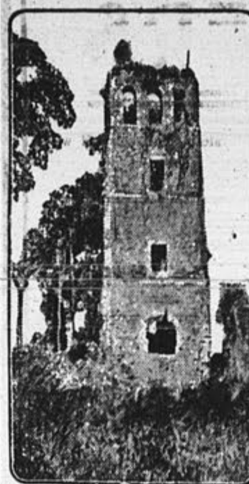
"Morgan's Tower," Old Panama.
