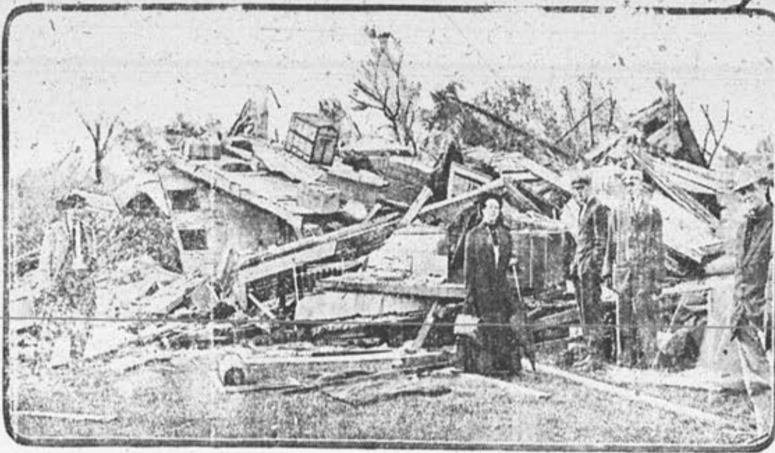
This shows all that was left of the residence of C. Kollmeyer by the terrible storm that swept Seward. The house was the oldest in the town.
