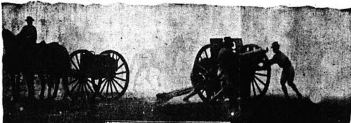
BATTERY IN ACTION
