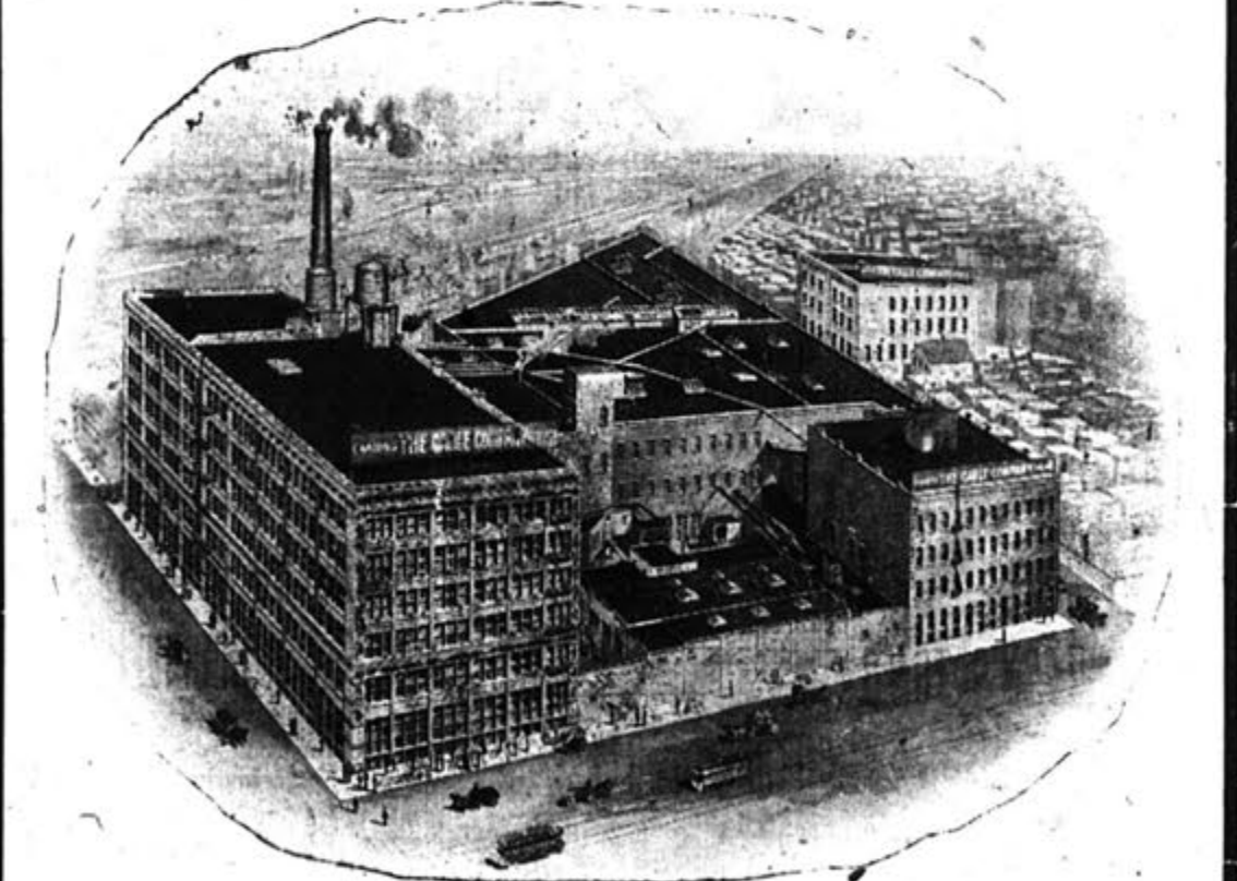
This photograph taken from a captive balloon. Photographic cuts of our other factories and buildings will appear in this space in subsequent issues of the "Mirror."
