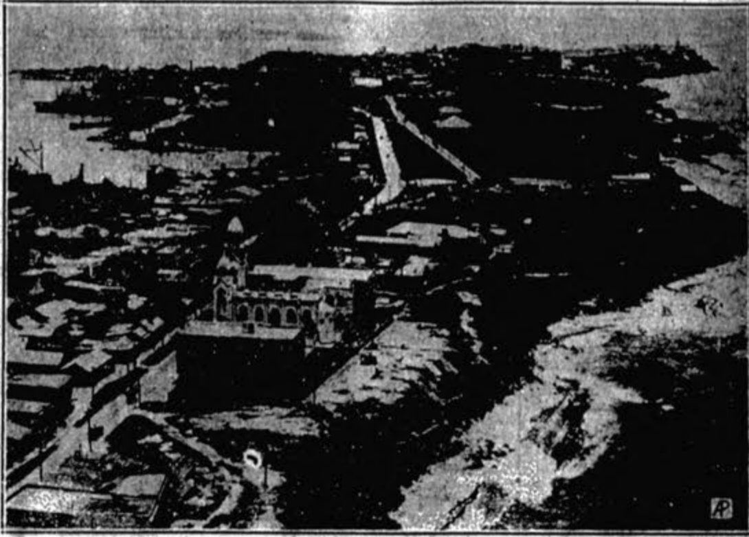
General view of the waterfront at San Juan, Porto Rico, which was swept by a disastrous hurricane. Tens of thousands of persons on the island were estimated to be homeless. Aid is being rushed to the island to avert the ravages of famine and disease.
