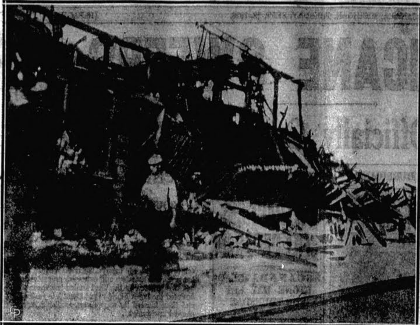
Struck by a terrific tornado which lashed its way through Rockford, Ill., this four-story cabinet factory collapsed, crushing and burying 100 workers in its ruins. This Central Press telephoto shows the wrecked building and part of the huge pile of debris, from which the bodies of victims were removed to morgues and hospitals with great difficulty.
