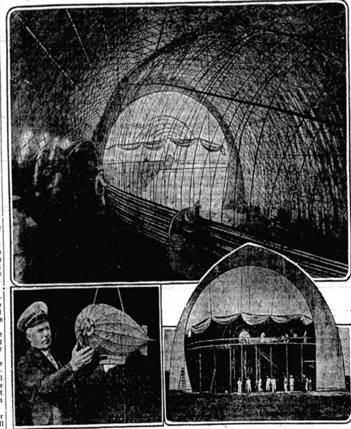
At the top is an interior view of the giant hangar where the hull of the City of Glendale is being constructed. Captain Thomas B. Slate, designer, is shown, lower left, with a model of the dirigible as it will appear when completed. Right is shown one end of the hangar and the nose of the ship in which the steam turbine will be installed.
