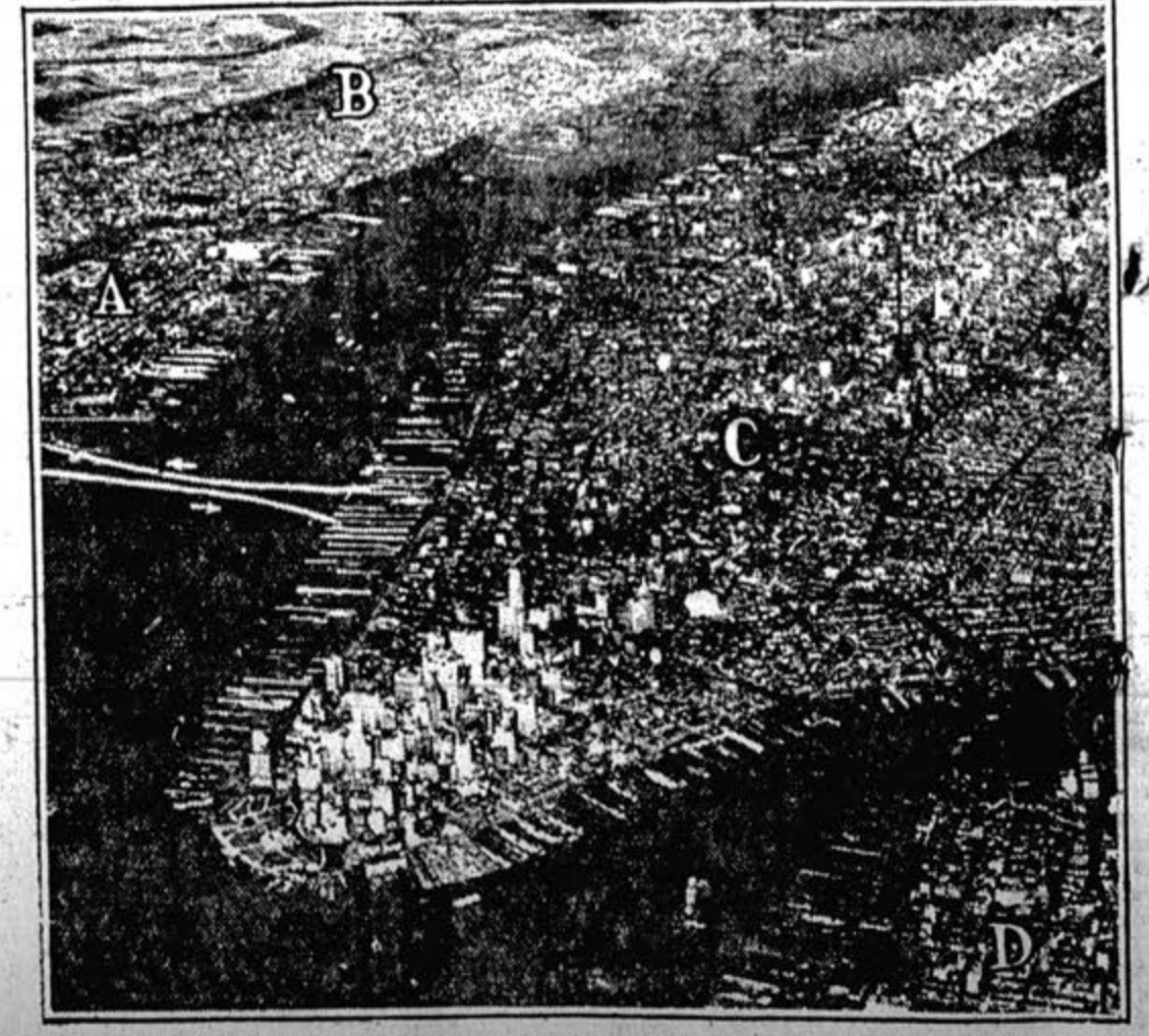
THE LINES ACROSS THE Hudson River at the left of this air photo indicate the location of the twin Holland $48,000,000 vehicular tubes connecting New York and New Jersey, just opened. The tubes afford New York relief from many troublesome traffic problems. The letters indicate: A, Jersey City; B, Hoboken and Weehawken; C, Manhattan; D, Brooklyn.
