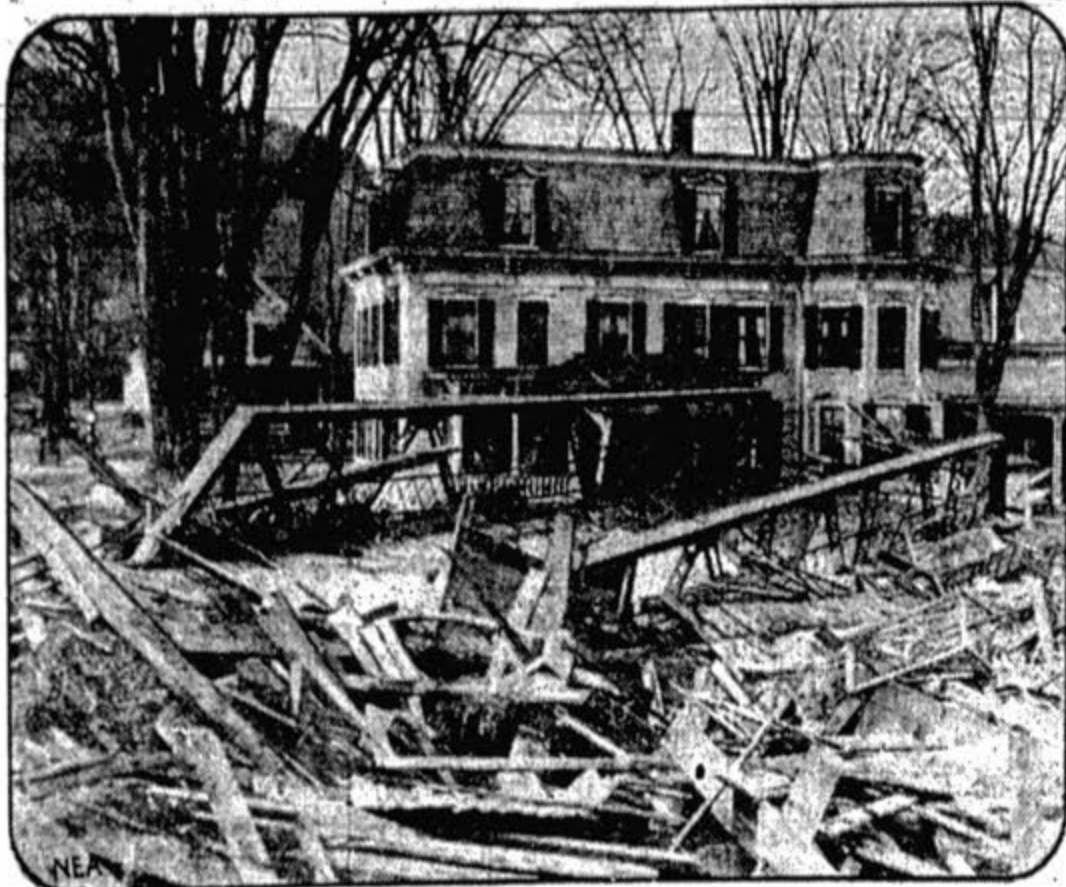
Occupants of this Montpelier, Vt., home found a badly smashed steel highway bridge on their front porch when they awakened the morning of the flood. Ever see anything like it before?
