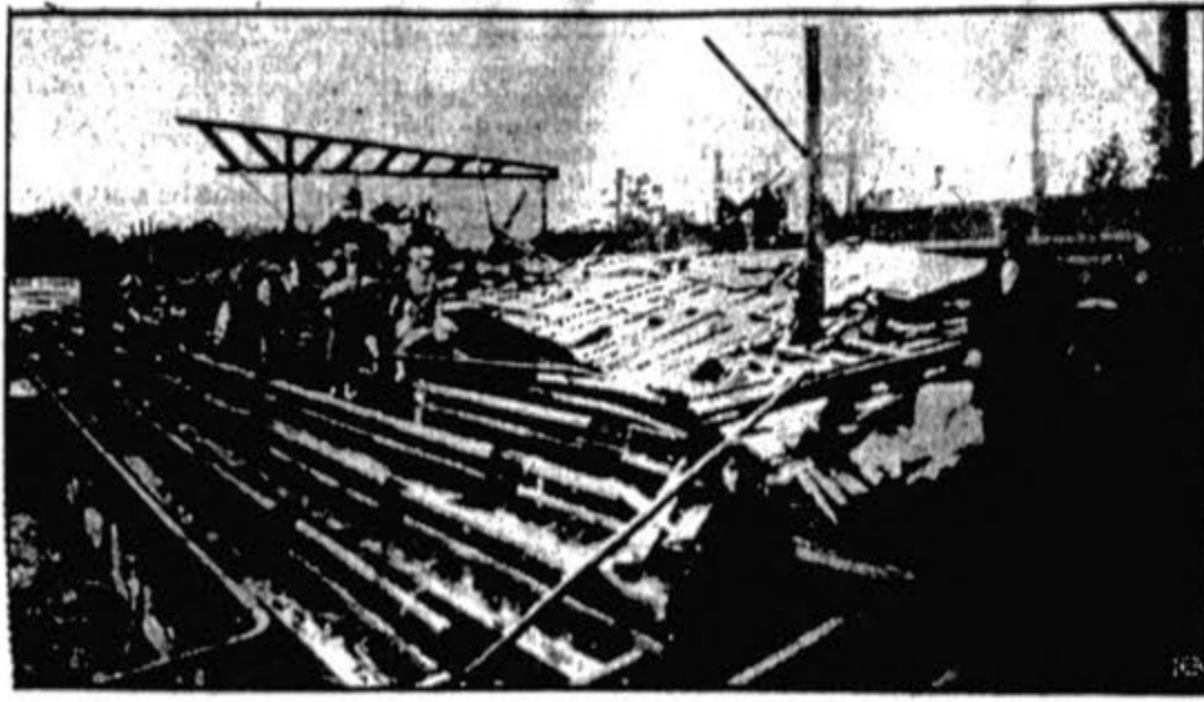
This is the wreckage of the Virginia League baseball grandstand at Norfolk, Va., which was blown down by a sudden 70-mile gale. Four fans were killed and 25 severely injured. Judge Keneaw Mountain Landis, high commissioner of the diamond, was watching the game in progress when the storm blew up, but escaped unhurt.
