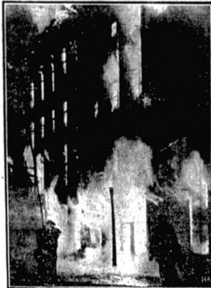
HERE ARE THE FLAMES consuming the Y. W. C. A. and the Hatch building in Bangor, Me., in the early morning fire which did $1,000,000 damage and threatened the entire business district. It raged for four hours before it was brought under control.
