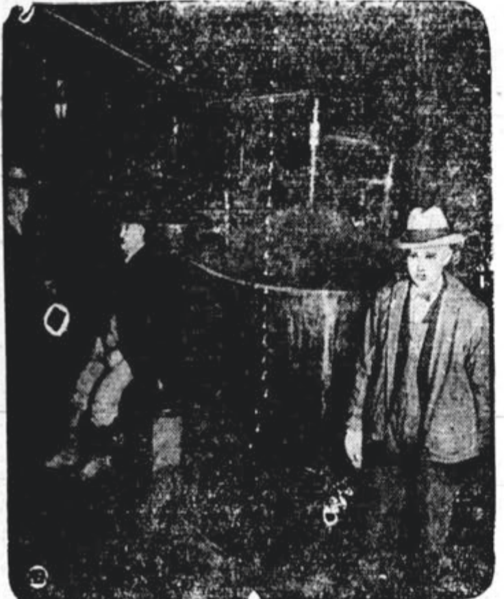
FIND STILL'S 200 FEET DOWN—An elaborate whiskey distillery in an abandoned lead mine, 200 feet under the surface, was raided by federal prohibition men at Picher, Okla. Four 1000-gallon stills were seized, and the raiders found the distillers had piped gas, water and electricity into the old mine and had an electric elevator to take them up and down.
