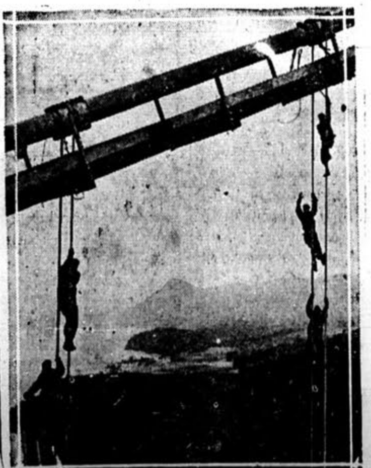
CELEBRATING END OF JOB—These men are cutting dikes 155 feet in the air because they have just completed the span of the new suspension bridge across the Hudson River at Peekskill, N. Y. It is the highest and longest suspension bridge in the world. Its main span is 1625 feet long. Its towers are 350 feet high.
