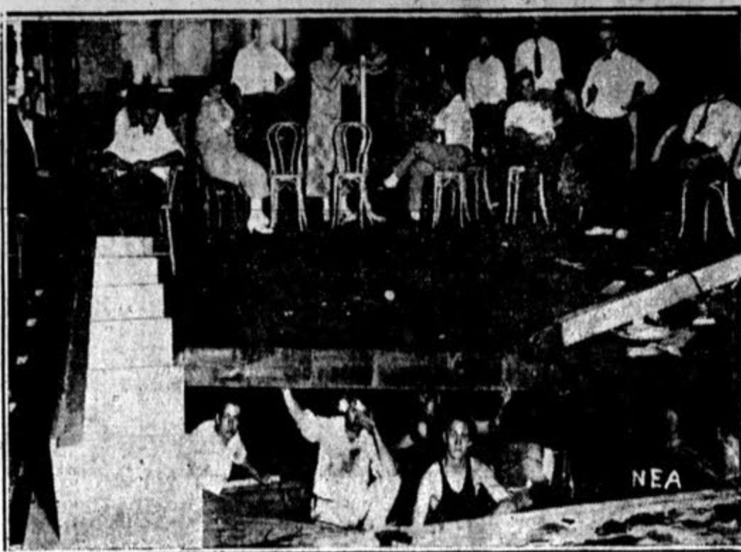
Eight persons were drowned near Buckeye, O., when part of a dance pavilion built over the water collapsed. The accident was caused by a beam under the floor breaking when the floor was crowded. Thirty persons fell through the floor into the water. In the picture men in a boat may be seen hunting for bodies.
