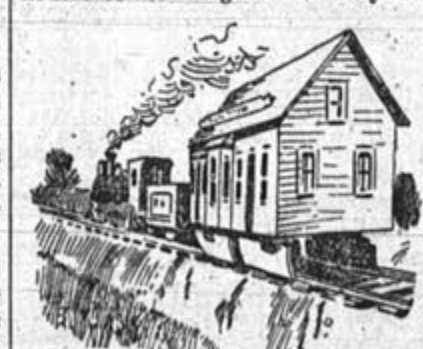
STATION ON SKATES. (Pulled from one End of Town to the Center by a Locomotive.)
