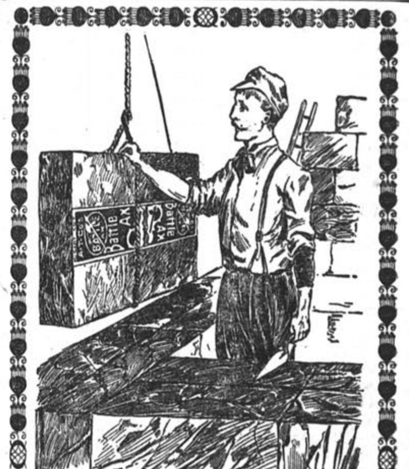
"A Good Foundation."
