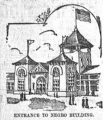
ENTRANCE TO NEGRO BUILDING.
