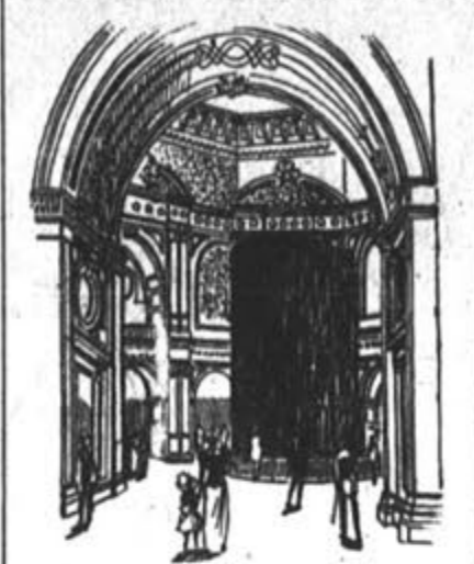
ROTUNDA IN GOVERNMENT BUILDING.
