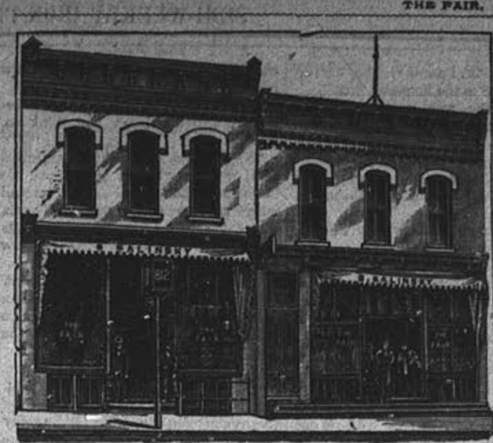
This Cut Represents the Fair Building. 812 AND 814 LUDINGTON STREET.
