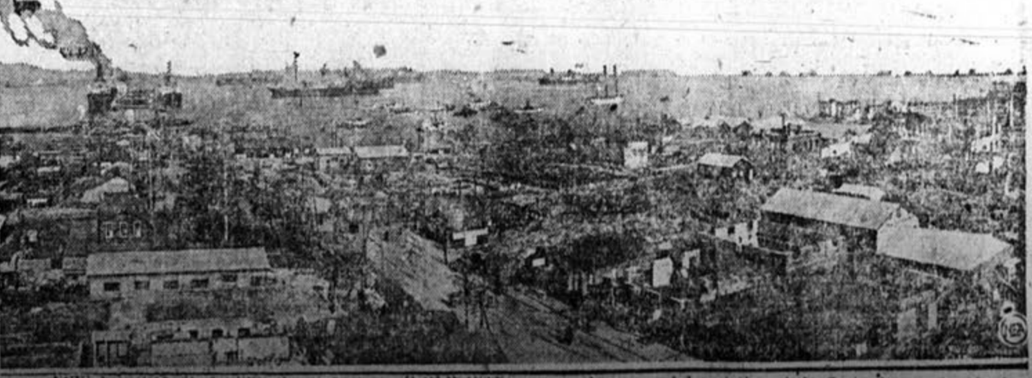
NEW YOKOHAMA RISES FROM RUINS OF OLD CITY—Out of the ruin and devastation of the September earthquake is arising a new Yokohama. Clusters of tiny Japanese bungalows and temporary office buildings are springing up on the sites where buildings were razed, and material is being rushed in from all parts of the world for a comprehensive program of business house building. All of the homes shown in these pictures except some charred hulks, have been built since the disaster. This picture was taken by the Admiral Oriental Line, American shipping company, whose buildings were also wiped out in the disaster.
