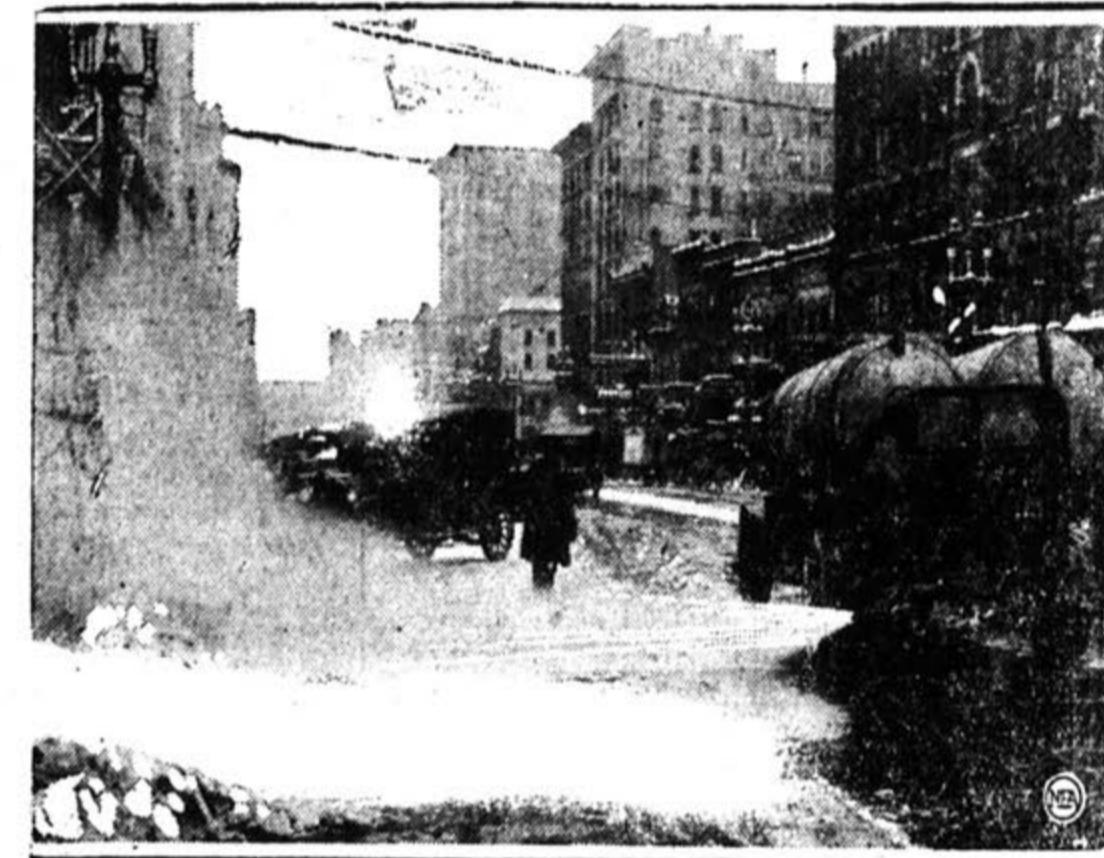
CONQUERING THE SNOW KING —In Salt Lake City they use hot water to flush the streets when snow impedes progress. Heating the water doesn't cost the city a cent, either, since it's piped from natural springs at 110 degrees Fahrenheit. Photo shows a municipal sprinkler pulling the fade-away act on a lane of the wintry staff.
