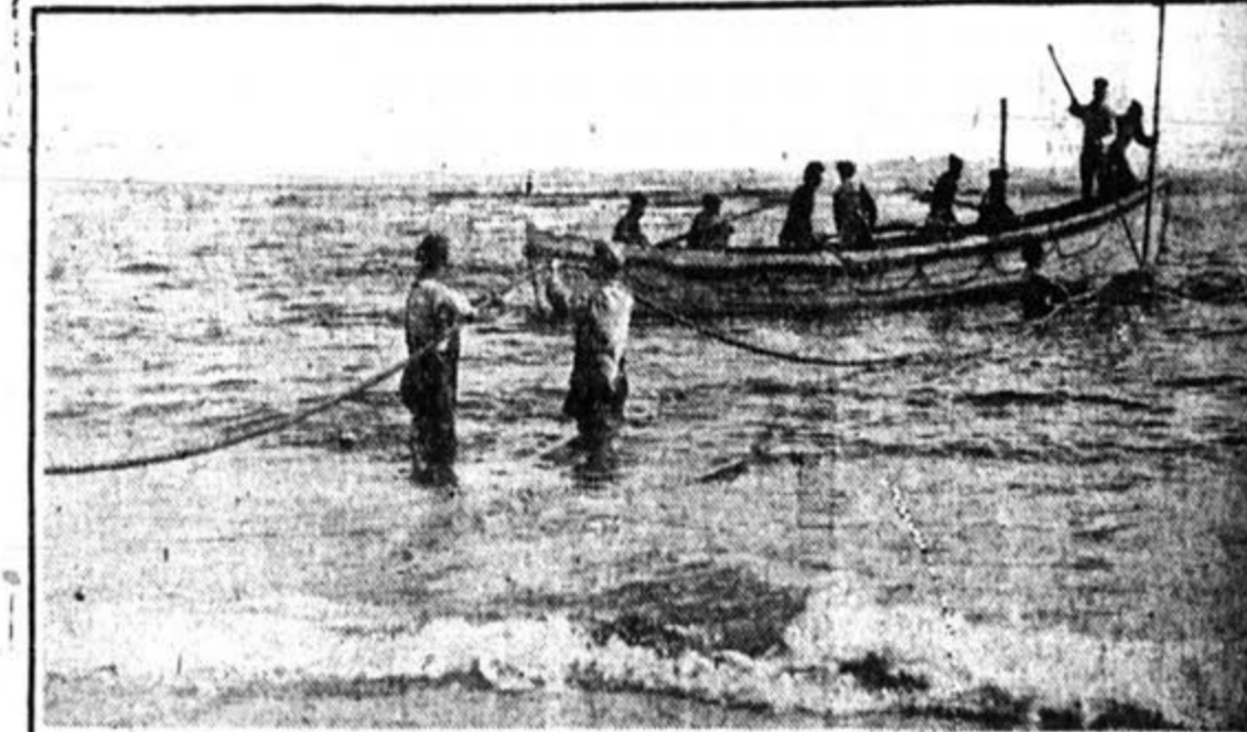
ANOTHER STRAND ACROSS THE SEA —Here is the start of the laying of the eighteenth cable connecting the United States and Europe at Far Rockaway, N. Y. Despite the increasing use of radio, popularity of the cable still grows. The new one will be the longest and fastest.
