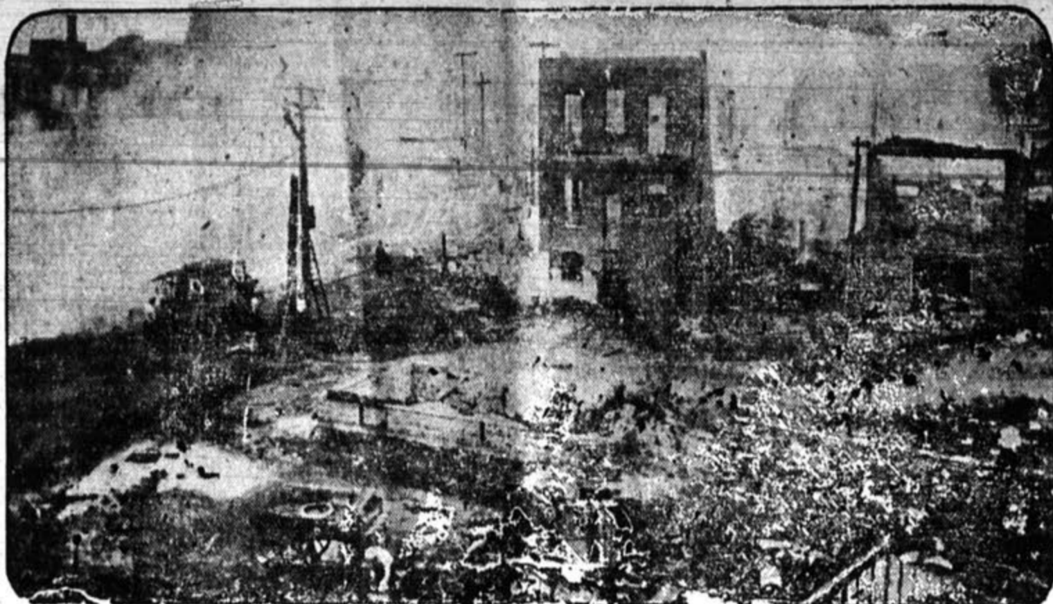
A view of Salamanca, N. Y., shortly after a fire causing $1,000,000 damage swept through the town. Business and residence sections suffered heavy losses and the city hall was destroyed as oil, gasoline and dynamite were ignited by the blaze.
