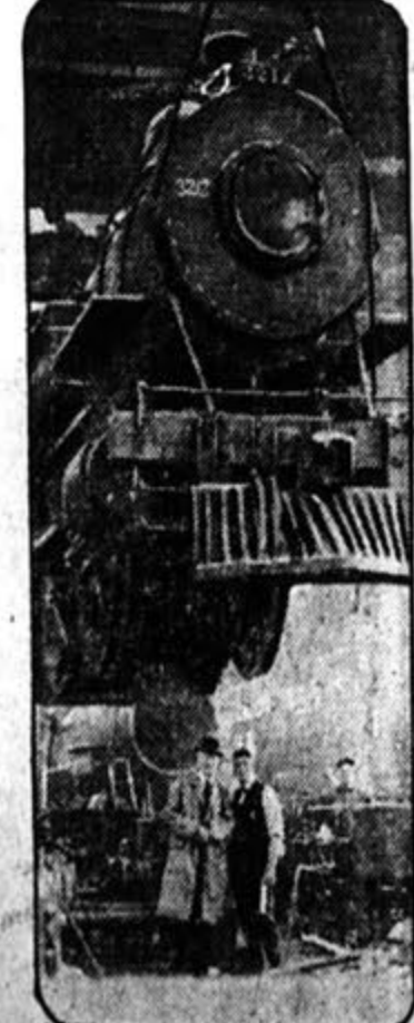
LOOK OUT, BELOW! —If a chain holding this 90-ton locomotive should break or a support slip, the men below might not appear so unconcerned. But they don't seem to worry much, for they are veteran employes in this railroad shop at Billerica, Mass.
