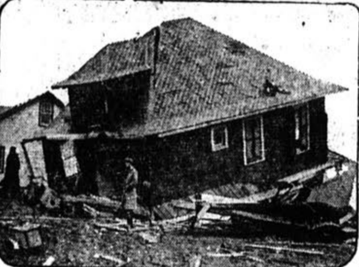
MORE EXCITING THAN THE MOVIE —Dr. and Mrs. Edwin Dudley returned from the movies and found their home at Sligo, Md., as it is shown here. A tornado had torn it from its foundation and turned it partly around. The nurse was dressing the baby when that happened but both escaped uninjured.
