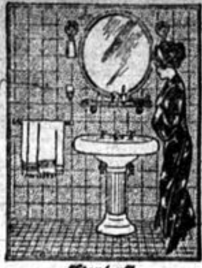
Standard Toilet Lavatory
