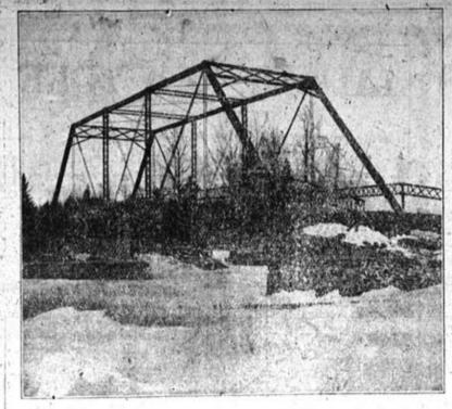
Cole Bridge, Masonville Township, 90-foot span on concrete abutments. Over the Rapid. Erected by the Joliet Bridge & Iron Company, Joliet, Ill. Upper Peninsula Agency; Menominee, Mich.
