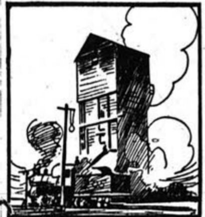
Getting Coal and Sand Supply.
