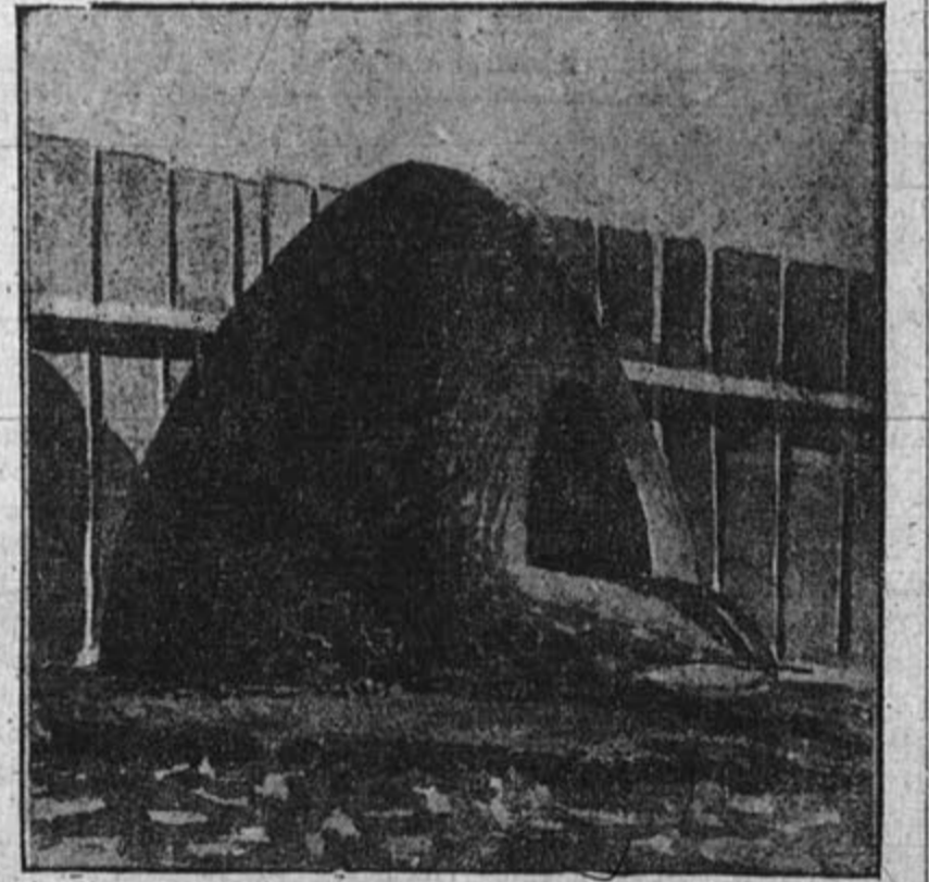
Although living within hailing distance of the United States, the Mexicans still cling to antiquated business and household methods. The picture represents an adobe oven, such as is commonly seen in Mexico. The one here illustrated was photographed in El Moro, near Trinidad, southern Colorado, a region given over to the Mexicans. While the bread or meats are prepared, the oven is filled with wood, which is set on fire, but burns very slowly. When it is thoroughly heated the fire is raked out, the food put in quickly and the door shut again. The baking is said to be very even.
