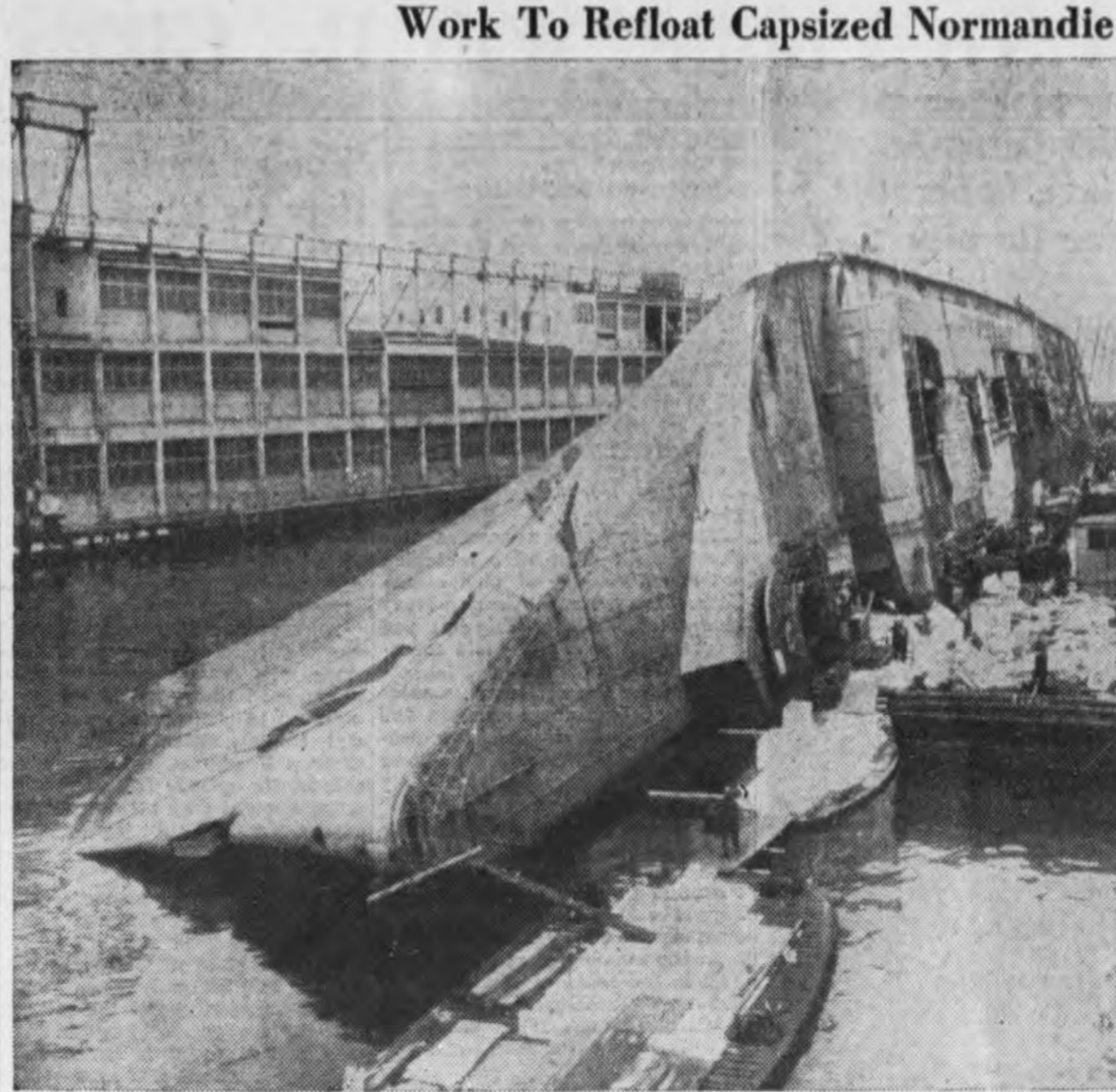
Preliminary work in raising the burned and capsized liner Normandie at its New York pier is under way. The Navy announced the job would take about a year. Barges and other equipment lie alongside the overturned giant in this picture.
