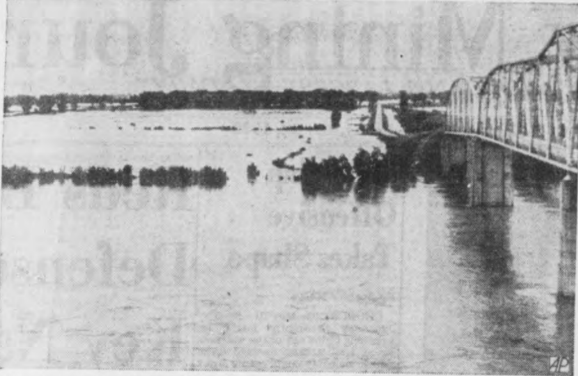
U. S. engineers termed this section of the Missouri river, at Nebraska City, Neb., the most vulnerable to high water, which was approaching near-record stages. Although dikes minimized damage at other points, the river spilled onto thousands of Iowa lowland acres and only trees and this bridge remained to mark its normal banks. No flooding has as yet occurred on the Nebraska side of the river.
