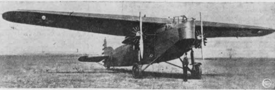
Atlantic LB-2, high-winged monoplane powered by two Pratt-Whitney "hornet" engines, used 1926-31.
