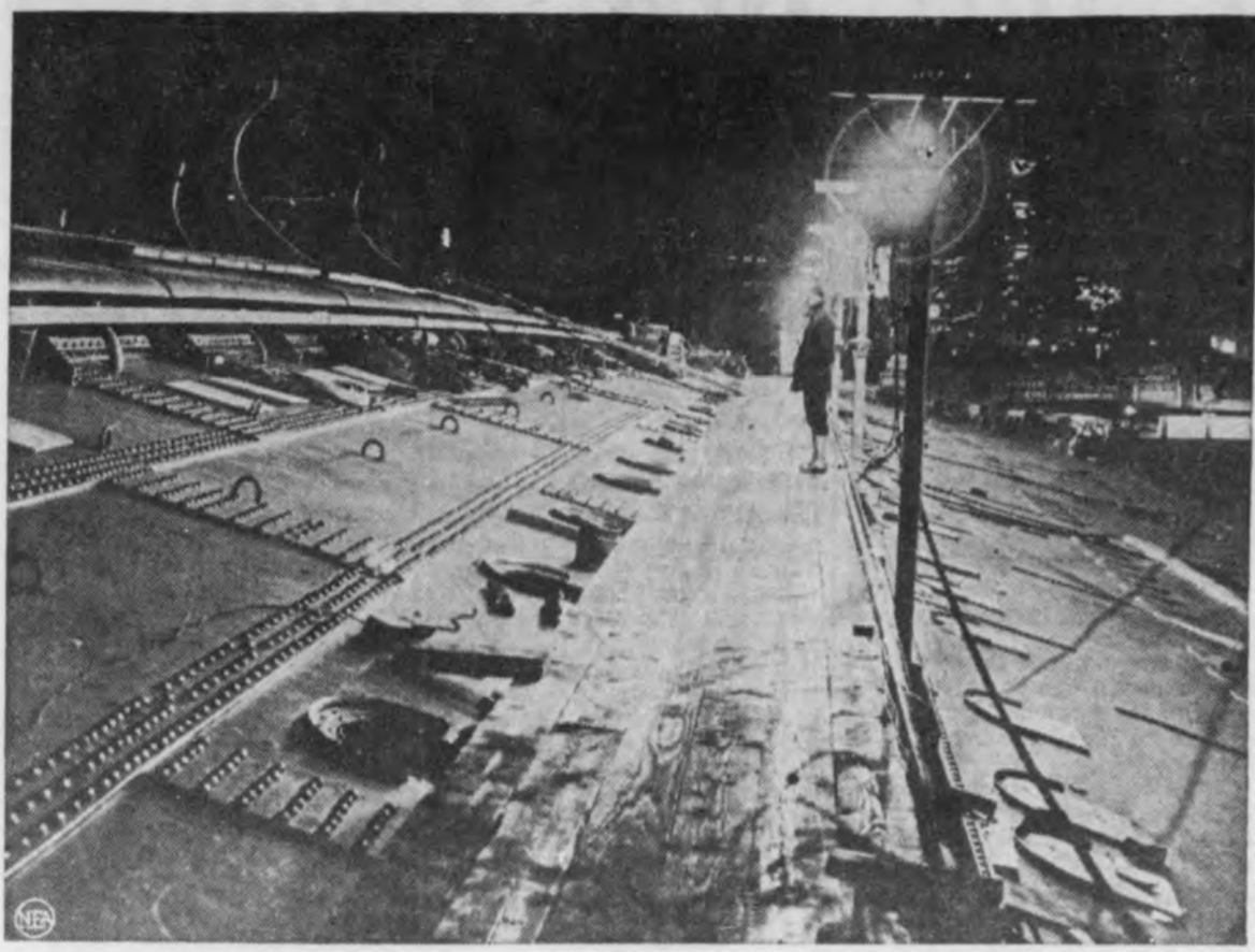
This isn't a sidewalk along a metal-surfaced street, but rather a lamp-lit board runway on the side of the U. S. S. Lafayette (ex-Normandie), built to aid in salvage operations of the capsized liner in New York.
