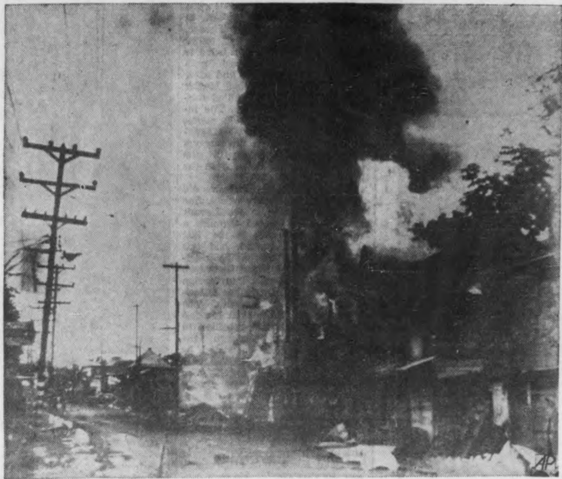
Burning buildings along Taft avenue in the Barrio Paranaque, Manila, Philippine Islands, roar testimony of the fury of the Japanese air raid of December 13, shortly after the war began. This picture is among the first to arrive in the United States from the Philippines since the start of hostilities in the Pacific. It came via Australia. (Associated Press Photo from U. S. Army Signal Corps.)
