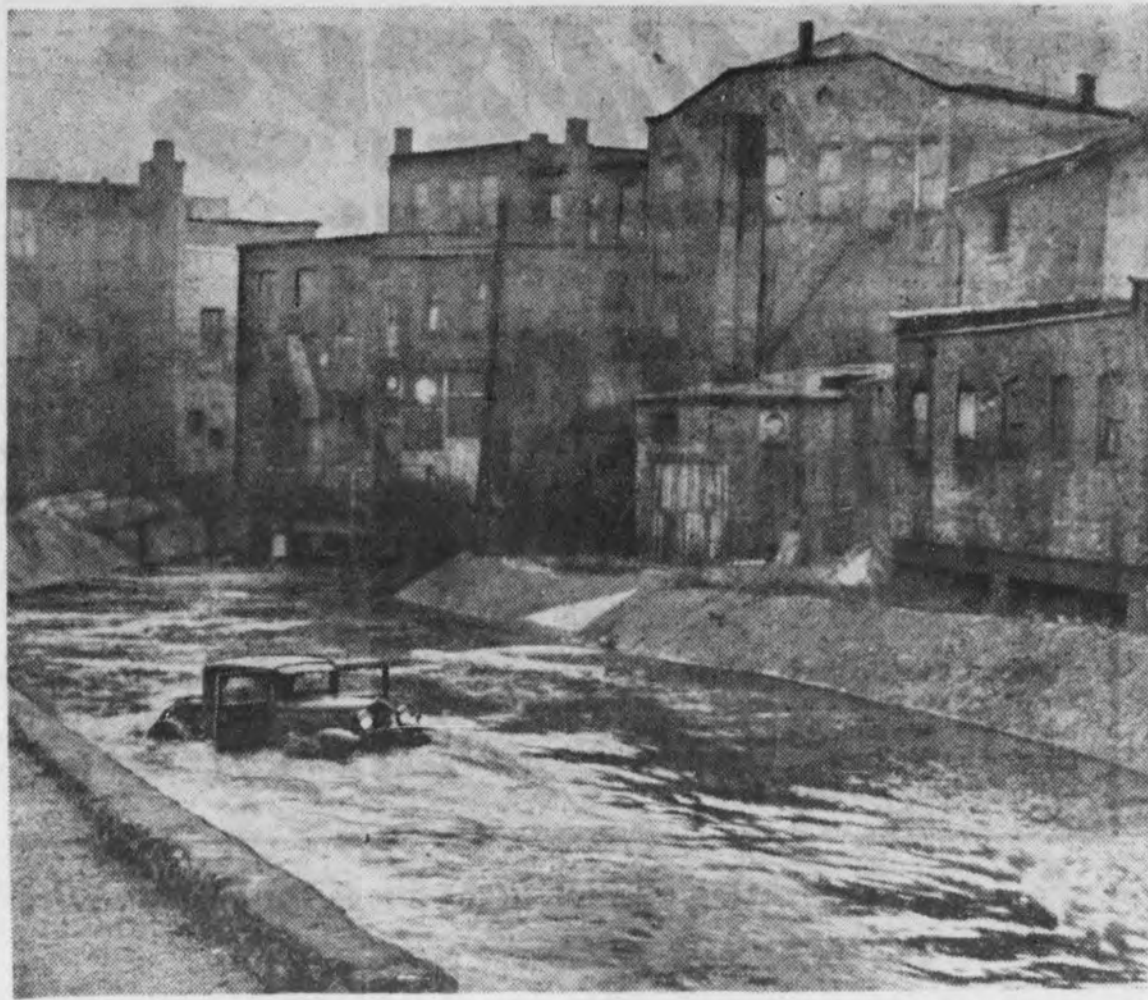
A car parked on the conduit of the Grand river in Jackson was trapped by the flood of water Tuesday. Normally the river flows through a concealed conduit but at this time of the year it frequently runs several feet deep over the conduit.
