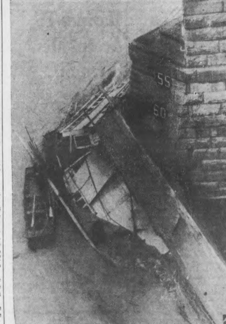
Only splintered wreckage (above), wrapped around a bridge pier, was above water minutes after the Ohio river towboat G. W. McBride crashed against the L. and N. span at Newport, Ky. Note men in small boat searching for bodies of 13 men and three women believed lost. (Associated Press Telegram)
