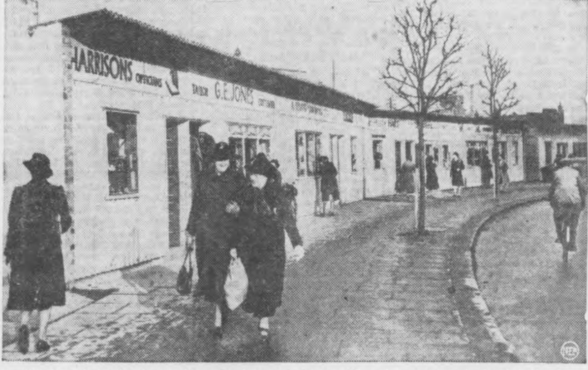
But Coventry today is marching ahead toward victory. Where homes were wiped out, better homes safer from bombs have been built. Emergency shops, like those above, neat and simple, have gone up where the bombers blasted the city's business districts.
