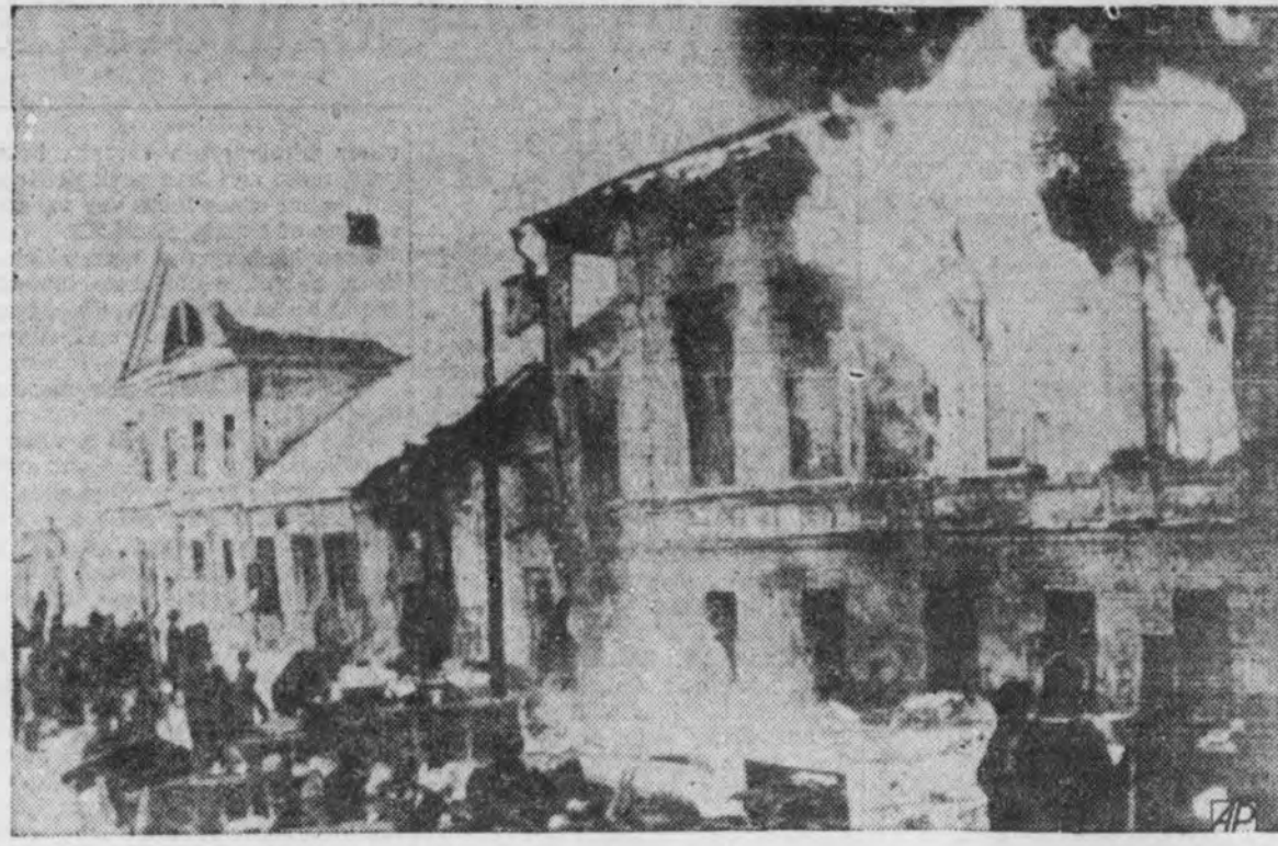
Flames sweep a building in Kalinin, Russia, as Red army troops enter the city, recaptured from the Germans in the Russian counter-offensive. This picture was sent from London to New York by cable. (Associated Press Telegram)
