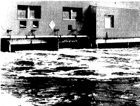
This is the area of the river where the foam water release at Manistique Papers, Inc. The foam is caused by protein in the water.
