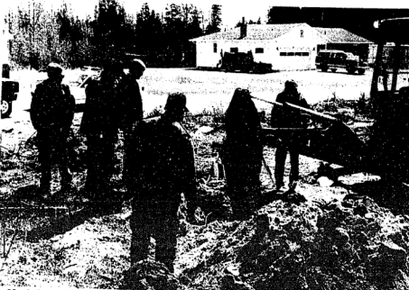
Manistique Public Safety officials, City DPW representatives, and Michigan State Police bomb experts excavate a vacant lot at the corner of Potter and Wilson Streets last Wednesday after dynamite detonation wires were found at the site. After the excavation, the bomb experts determined that no live dynamite was still in the area. Dynamite charges had been used several years ago when sewer lines were put in the area, according to Public Safety Lt. David Peterson, and the lines were simply left behind.
